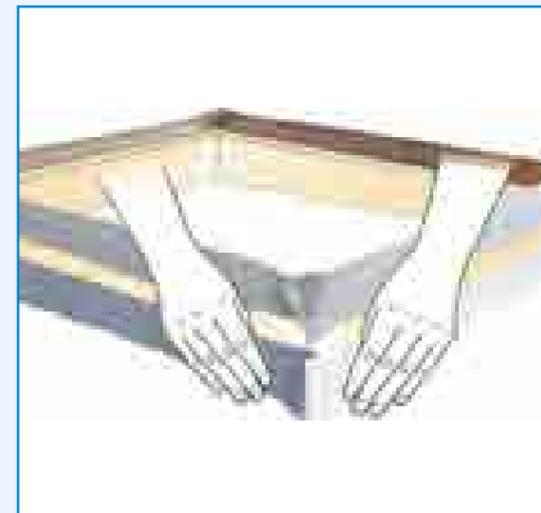
3 Now attach the exterior IsoWindow F1 tape (white and black) to the lower side (outer side) of the window frame in the same way. Once the tapes have been appropriately attached, the window frame can be lifted into the window opening. After installation fill the gap around the window with foam or with insulation material (e.g. IsoWindow Insulating Rope, IsoWindow Soft Cell Foam) and trim back as necessary.
