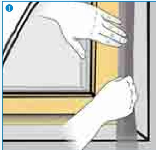
1 Cut the window tape with approximately 12cm excess in length. Pull off the backing paper from the adhesive strip and carefully press it onto the window frame, applying firm pressure either by hand or through the use of a roller.
